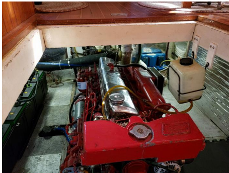
Engine room from saloon deck looking aft
